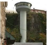
as a hydraulic steel and wood elevator, it was replaced by an electric elevator in 1955. The elevator is 130 feet high.
